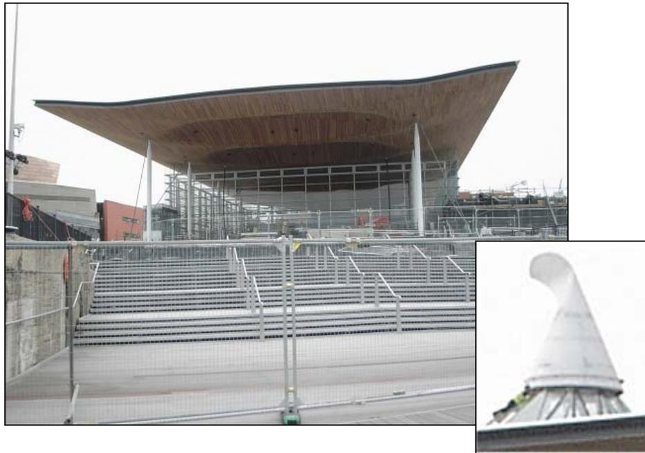
Figure 1. View of the Senedd building, Cardiff (Wales, United Kingdom) with rooftop funnel for enhanced natural ventilation (inset)
